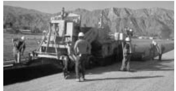
Top Left: Employees monitoring air quality Hanson Aggregates Mid-Pacific, Inc.
