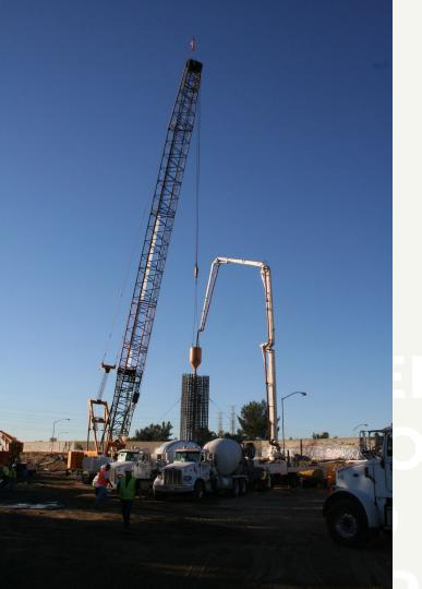
We can also encounter combinations of equipment, such as trailer pumps supplying concrete to boom pumps or a boom pump's boom connected directly to another boom pump.
