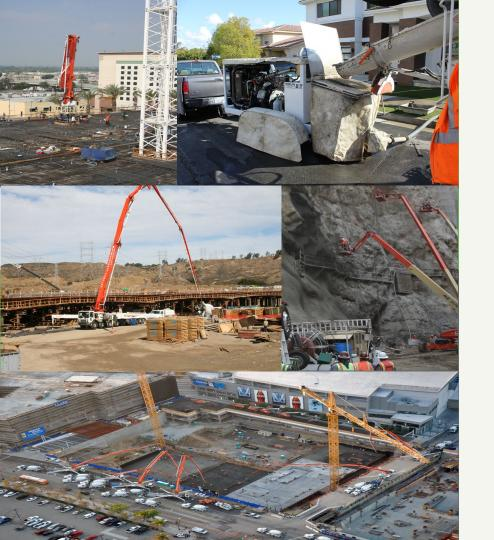
It has been estimated that 70% to 85% of ready-mix concrete is placed utilizing pumps.
